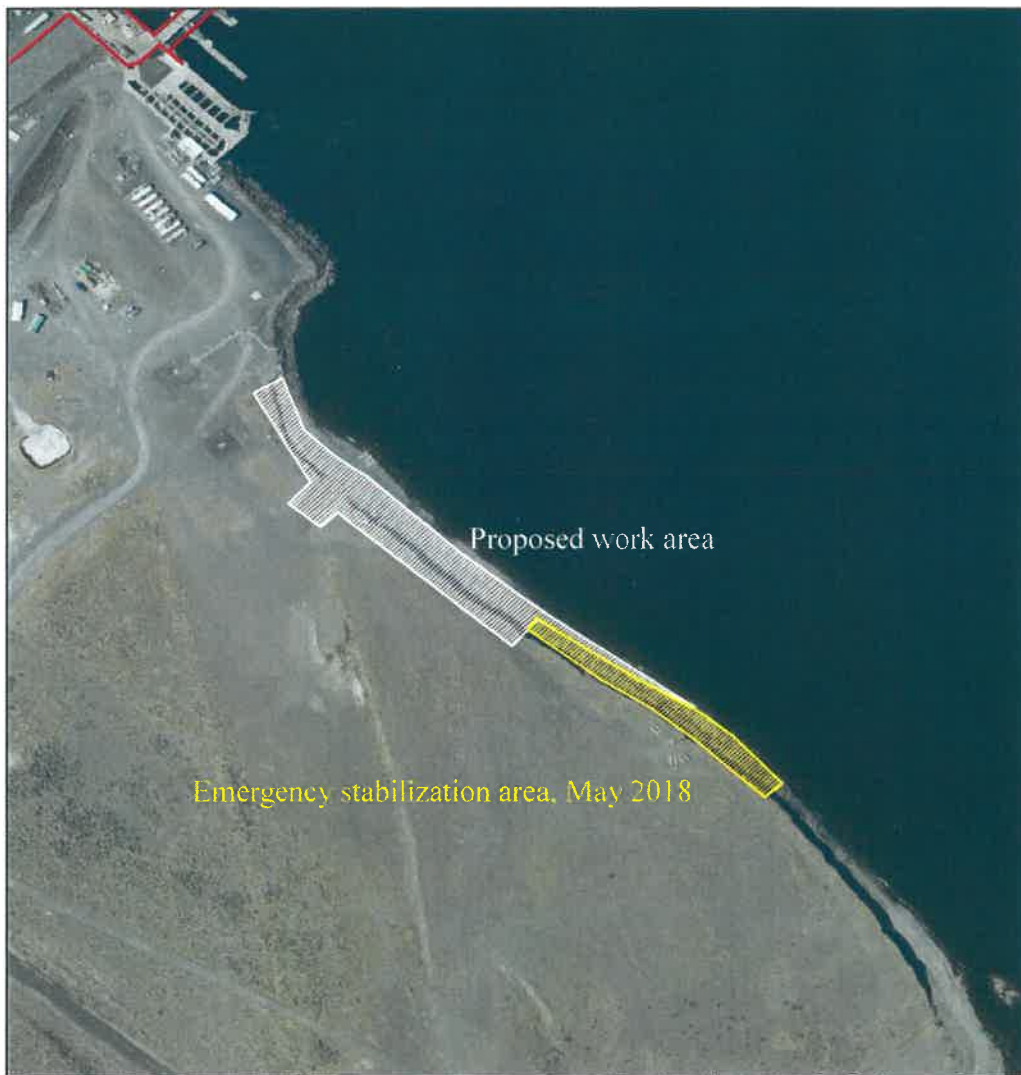
Figure 1 Wanapum Dam Right Bank Armor Project.
